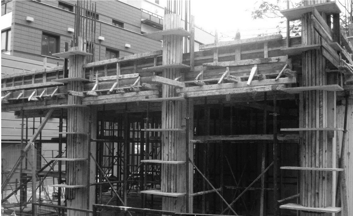
formworks cutted by laser-cutter, custom-made for the construction of the reinforced concrete columns
